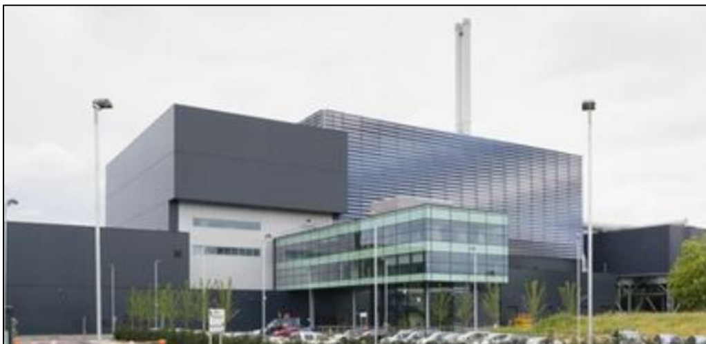
figure 2: Then Energy from Waste plant
