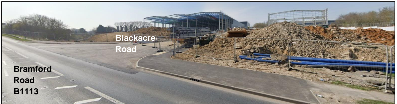
figure 3: Blackacre Road and view towards Port One [March 2022]
